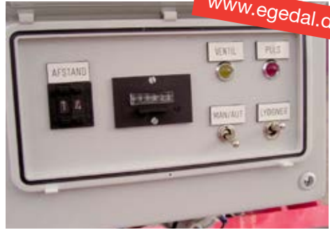
Setting of plant distance
